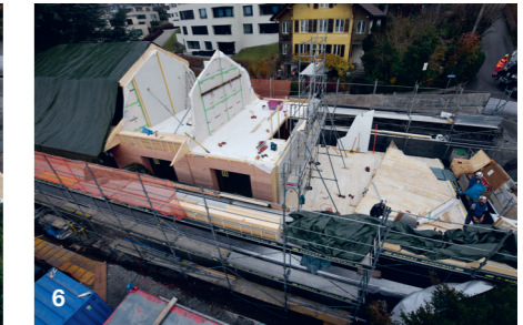
6 The timber construction is then erected on top of this as usual.
