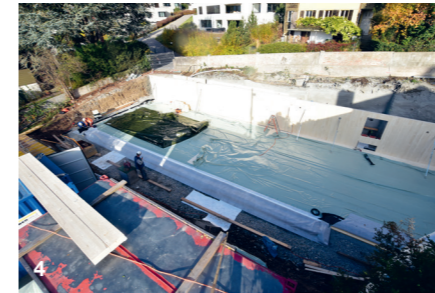
4 The walls in the basement are made of cross-laminated timber panels.
