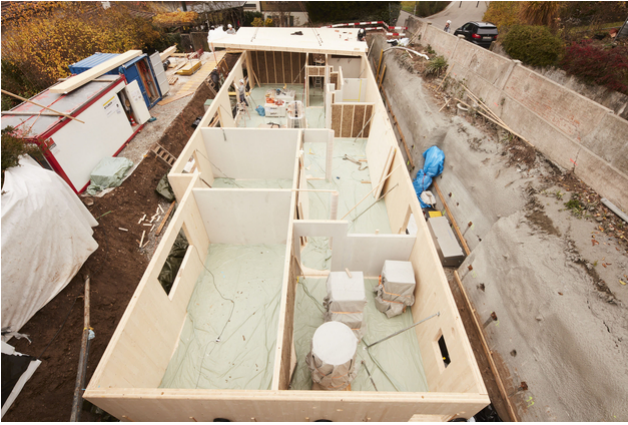
Basement during the construction phase
