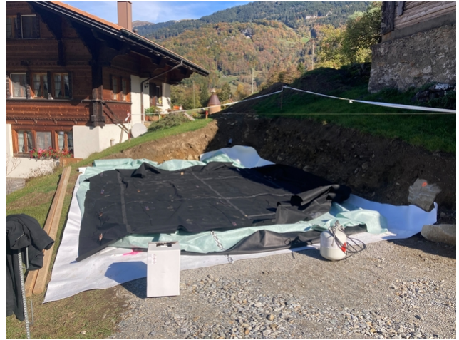
Waterproofing and moisture monitoring is ready
