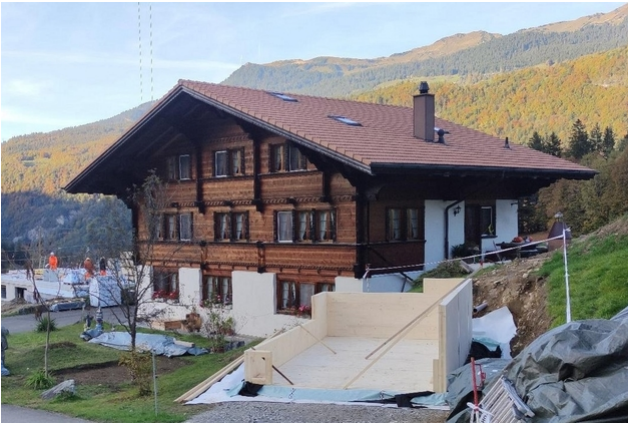
Cross laminated timber boards are grouted
